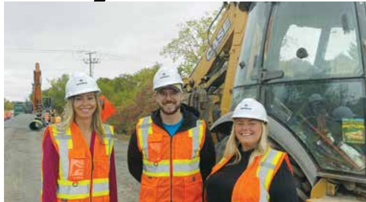
Gatineau Mayor Maude Marquis-Bissonnette, Aylmer Councillor Steven Boivin, and Deschênes Councillor Caroline Murray on the construction site for Phase 1 of the repaving and reconfiguration of Lucerne Boulevard.
